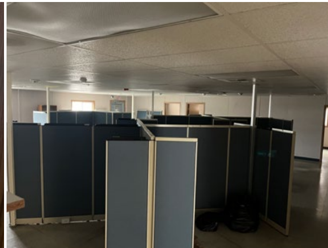
Open cubicle area
