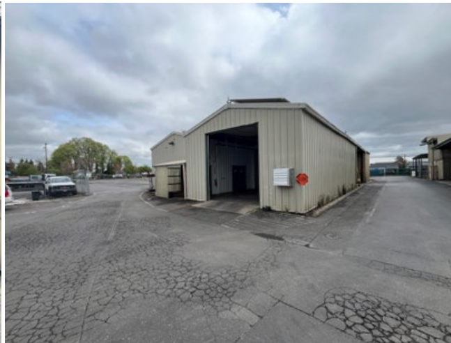
Warehouse west view
